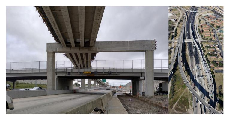
The IH-30 direct connector allows the traffic headed east on IH-30 to connect with the IH-35 Managed Lanes headed North, crossing over the General Purpose Lanes and Luella St. It is an 18-span bridge with an S-shaped layout. The design involved the widening of an existing structure and the design of a variety of pier typologies.
